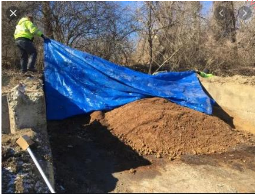
Figure 3.3.1.2.1: Typical impermeable membrane used to dry store topsoil on site.
